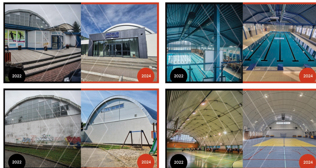
Before and after: upgrading the sports facilities in Luban
